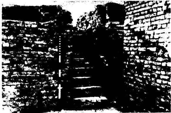
Fig. 67 A stairway leading to an upper floor in a Mohenjo-Daro house.
